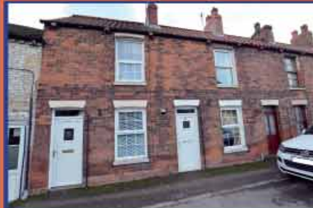
4 Main Street, Seaton £97,500 - EPC F Having undergone a huge transformation. Absolutely stunning country cottage
